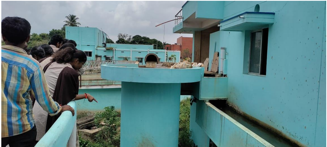
Fig: 1 Source of water supply from Salmalkot
